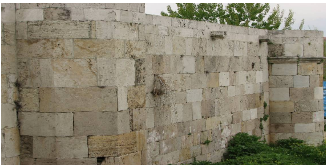
Fig. 57: The Well-cut Stone Blocks on the Outer Walls of the Courtyard
