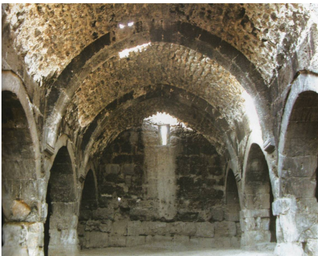
Fig. 56: The Pointed Arches and Barrel Vaults in the Shelter (Bayhan 2007: Fig. 14)
