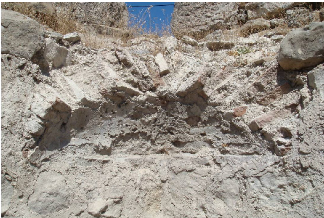
Fig. 13: The Brick Squinch from Room C
