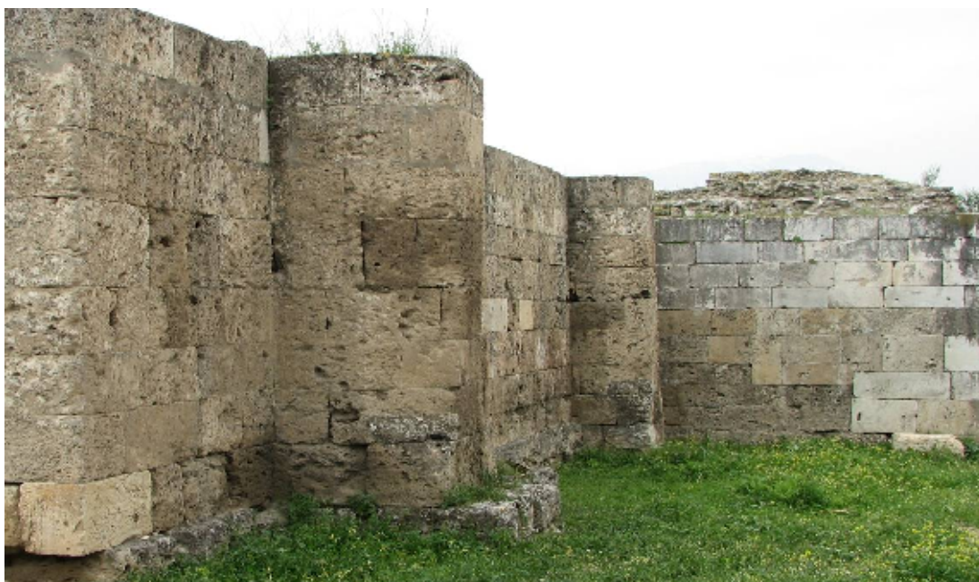
Fig. 55: The Polygonal Buttresses on the Western Outer Wall of the Shelter
