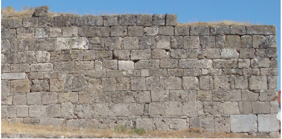
Fig. 33: The Variation in the Stone Block Sizes (the Western Outer Wall of the Shelter)
