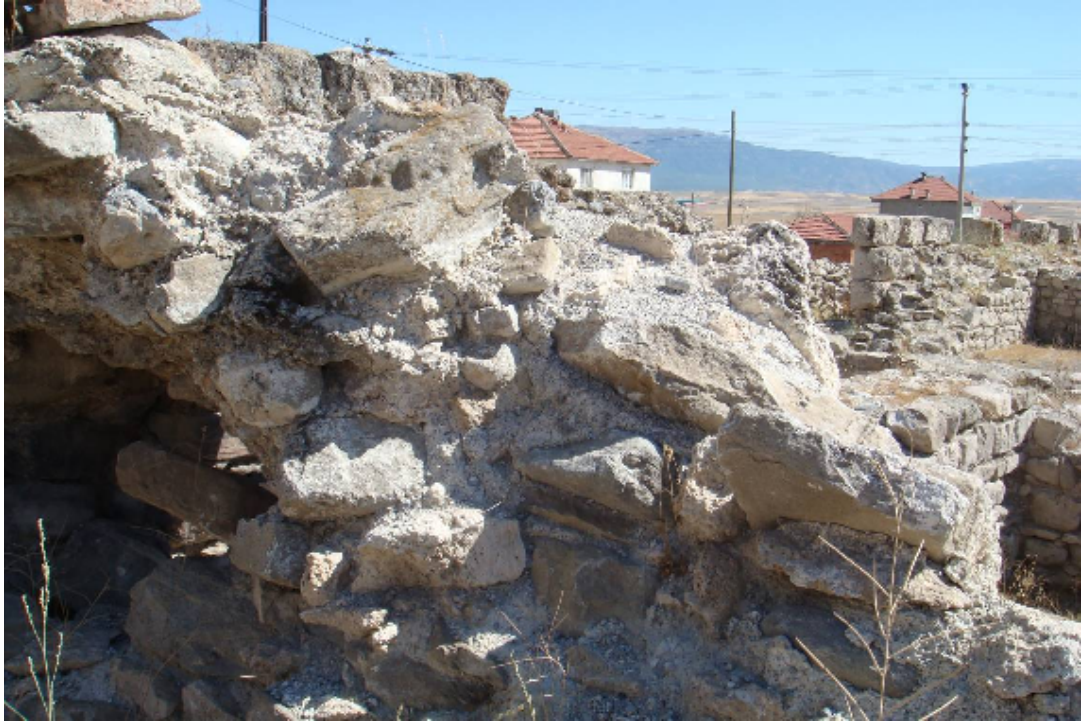
Fig. 32: Mortar with Pebbles and Cobbles (the Northeastern Corner of the Courtyard)
