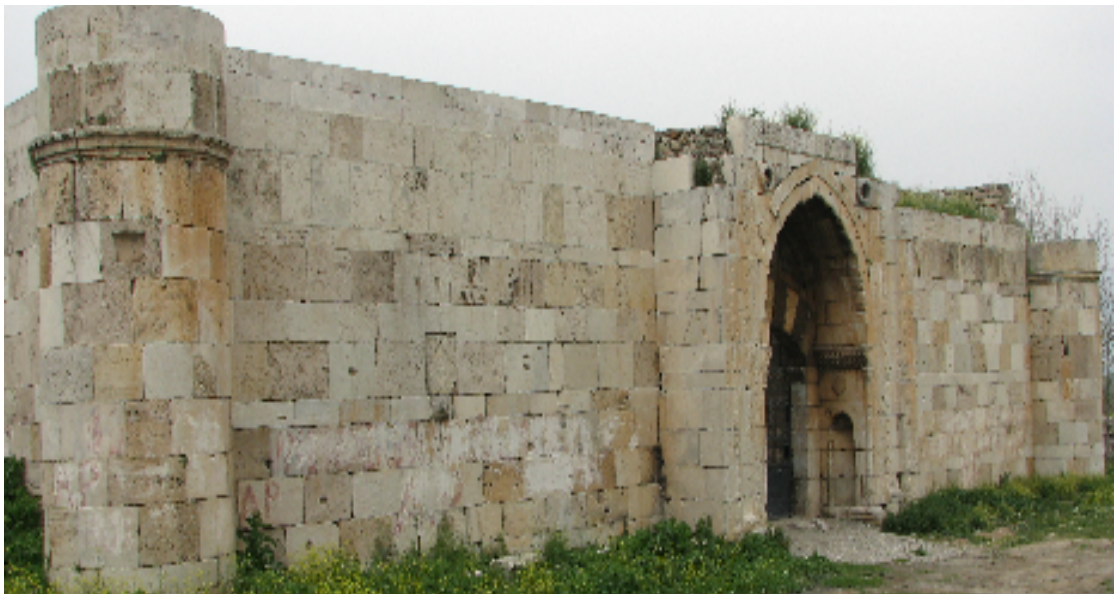
Fig. 48: The Cylindrical Buttresses of Akhan
