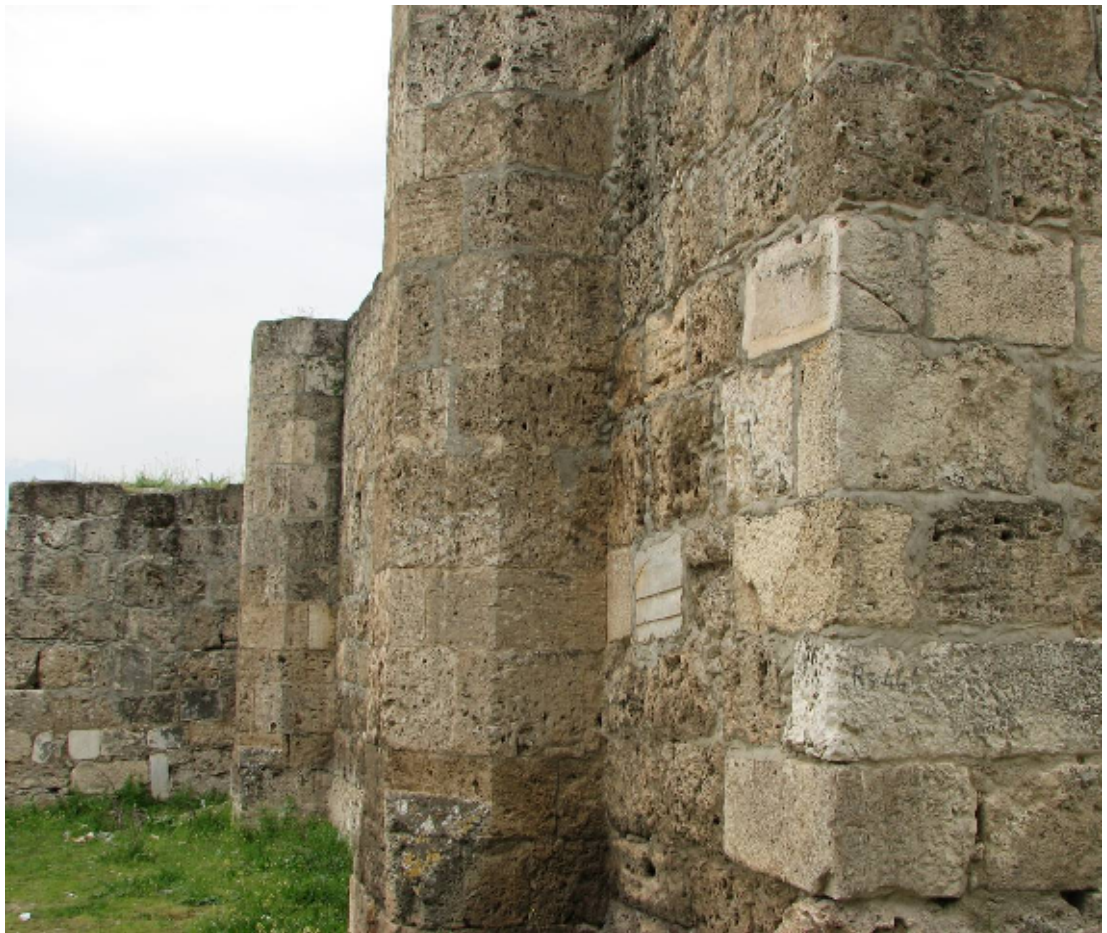
Fig. 54: The Polygonal Buttresses on the Eastern Outer Wall of the Shelter
