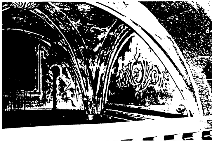
Figure 27 The stone ribs of the cross vaults and the plaster decorations
