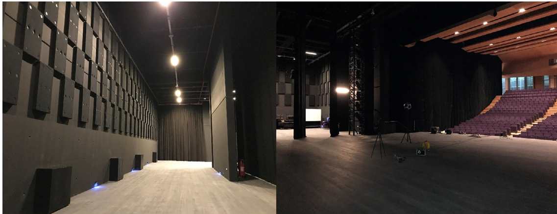
Fig. 7. (On the left) back stage with checkboard pattern mineral wool panel application on upper walls and over ceiling, (on the right) drama theater house dividing curtains in use, in stage field test configuration, side stage walls with checkboard pattern mineral wool panel application.
