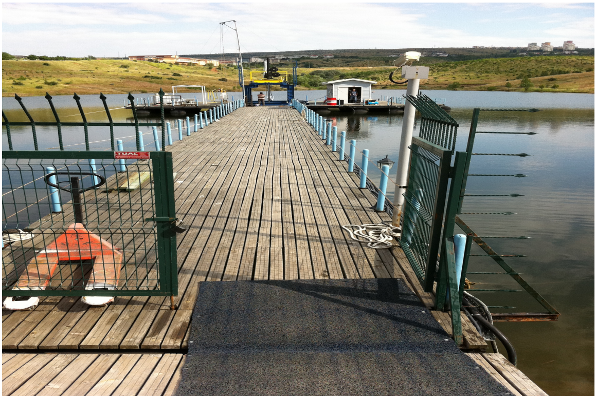
Figure 6.2: Bilkent Lake Facility
