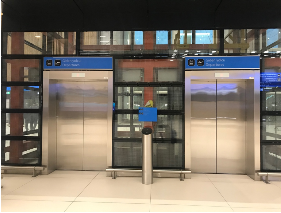
Figure F.5. Elevators (taken by the author, 2019).
