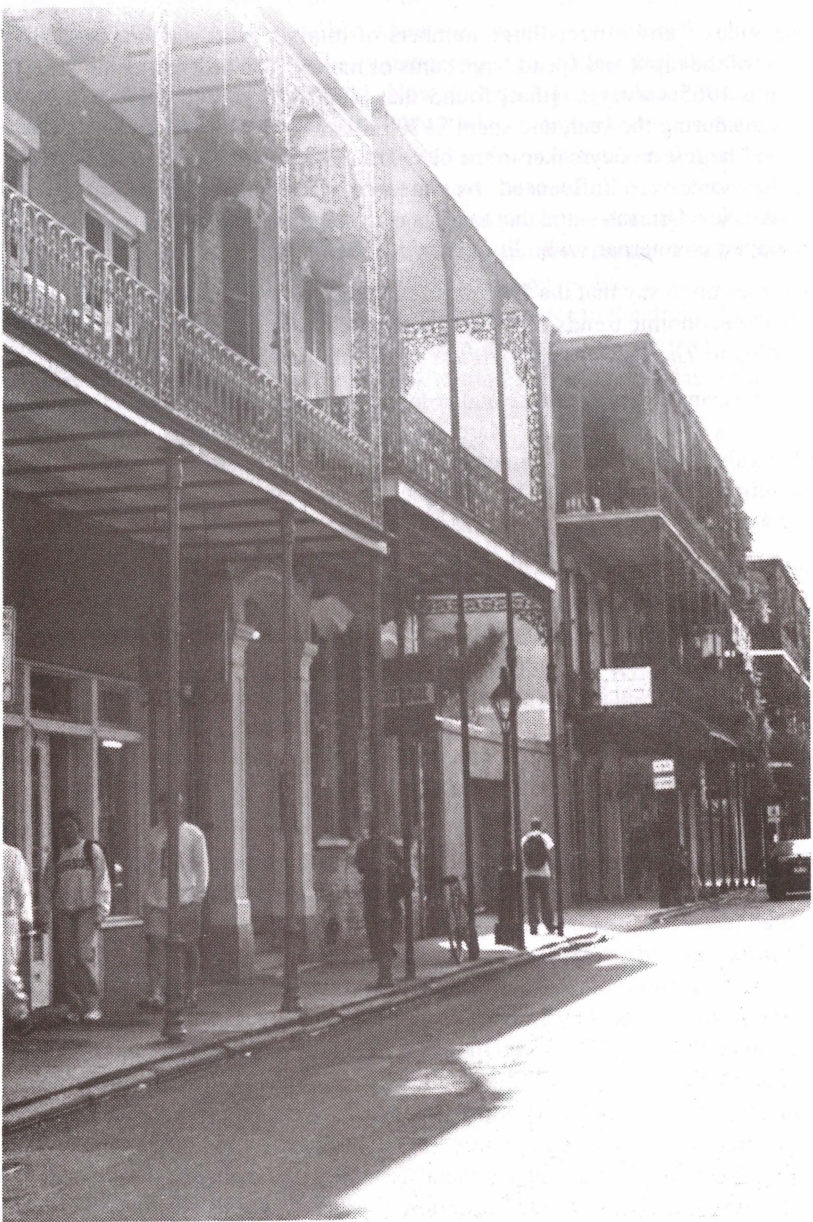
Figure 3. Spanish details on French Quarter building. Photograph by Reha S. Erzurumlu.
