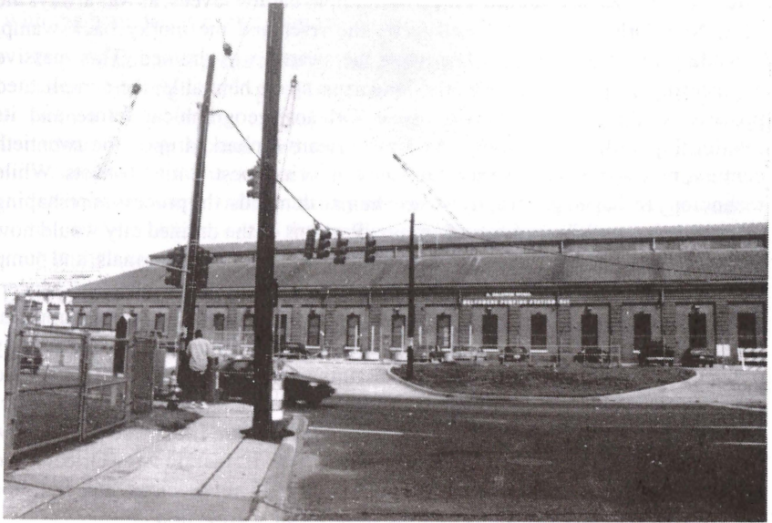
Figure 1. Baldwin Wood Pumping Station. Photograph by Reha S. Erzurumlu.
