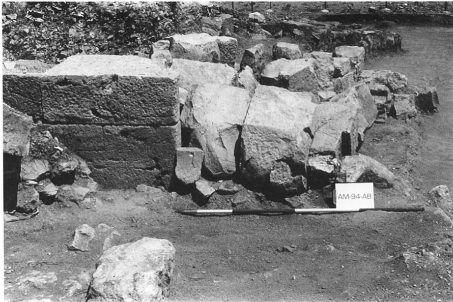
Fig. 43. Amorium. Lower City gate: collapsed lintel. (Courtesy C.S. Lightfoot)
