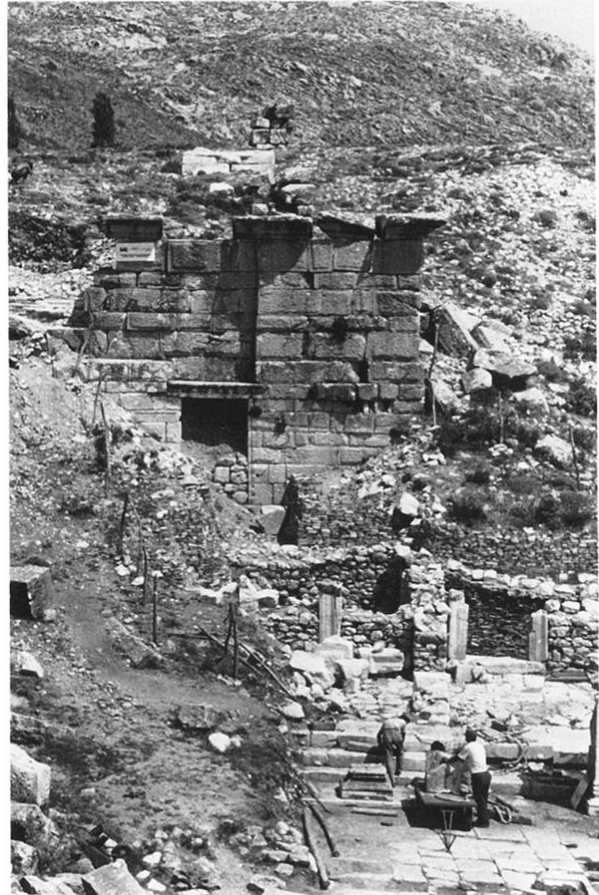
Fig. 32. Sagalassos. Partial view of a Roman bath building beside the Lower Agora, at close of the 1994 season. (Courtesy M. Waelkens)
