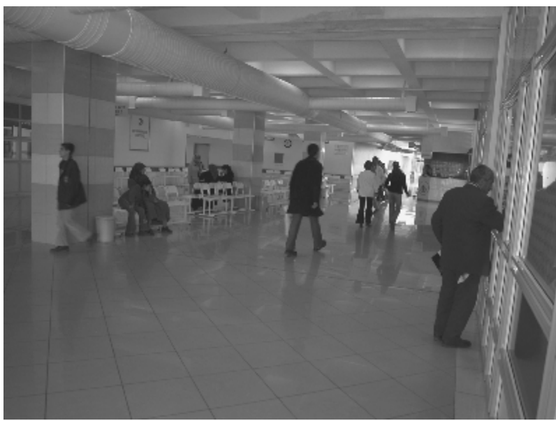
Figure 4b: Dicle University Polyclinic Circulation Corridor
