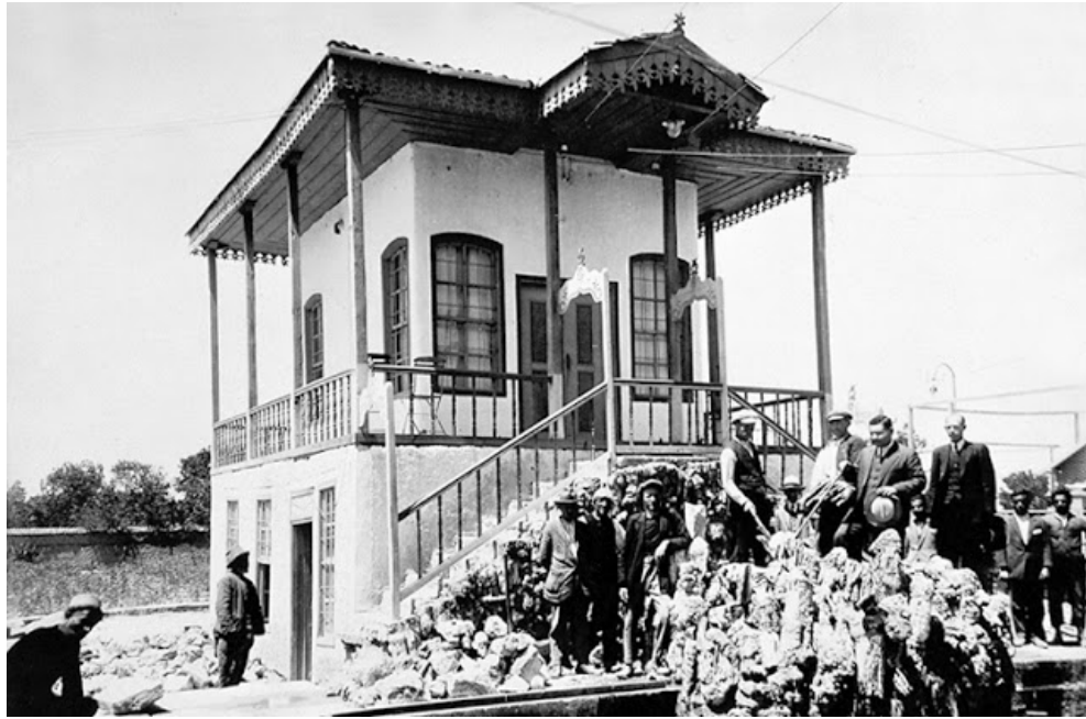
Figure 3.7: Maintenance and construction of waterfall on site (Source: Konya Metropolitan Municipality Public Work's Archive.)
