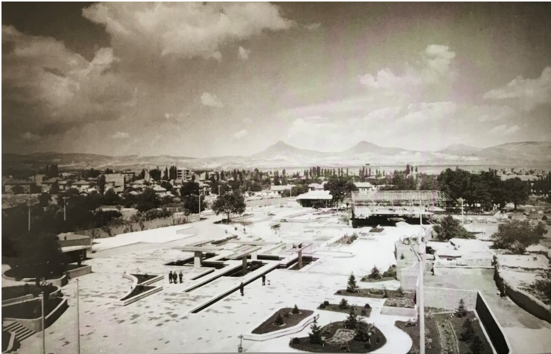
Figure 4.5: Culture park and fair construction before the opening; exhibition center was not completed yet (Source: Konya Ticaret Odası, Geçmişten Günümüze Konya Fotoğraf Albümü , Anadolu Ofset, 2018.)
