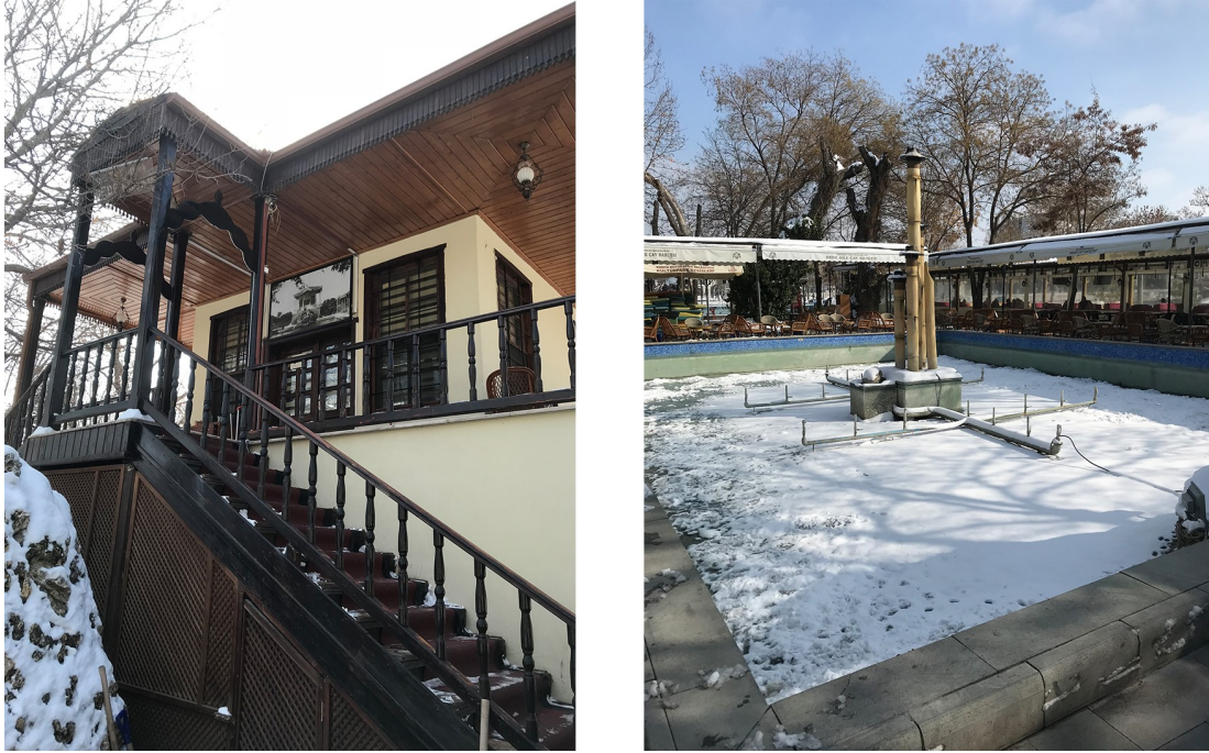
Figure 5.7: Dede Bahçesi Mansion and the pool was rebuilt in 2008 (Source: Photograph by the author, 2018.)
