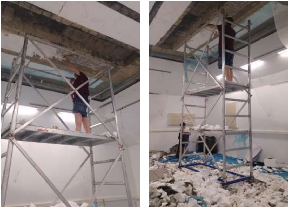
Figure 11 and Figure 12. EPS16 changes with EPS10 (by Erdemli)
