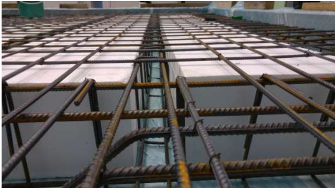
Figure 9. General view of iron reinforcement of girders and EPS block fillers (by Erdemli)
