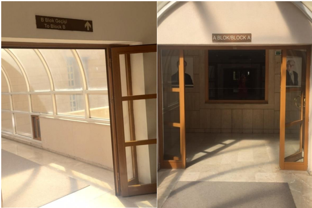
Figure 15: The bridge between A block and B block
