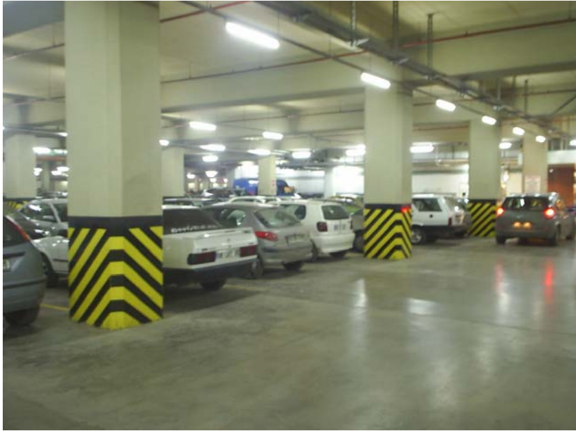
Figure 4. Closed parking area in Akköprü Migros Shopping Mall
