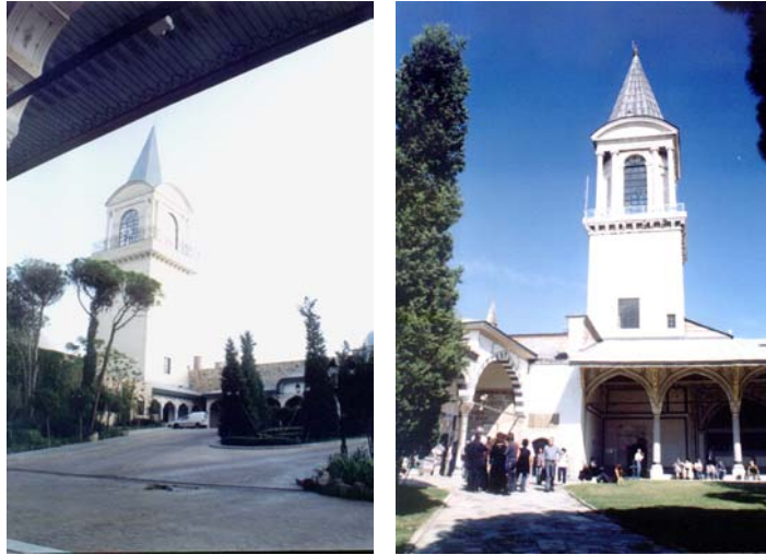
Figure 4.6 Panorama Tower on the left and Tower of Justice on the right.
