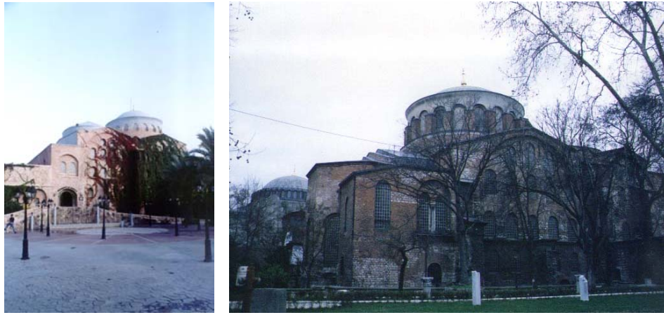
Figure 4.15 Disco-restaurant complex on the left and Hagia Irene Church on the right.
