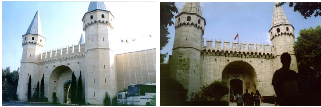
Figure 4.3 Hotel entrance on the left and Babüselâm on the right.
