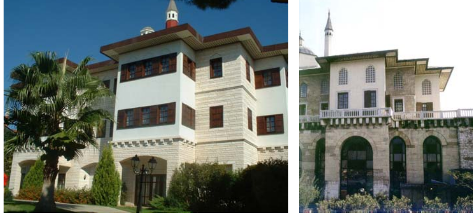
Figure 4.17 MNG House on the left and Basket Weavers Kiosk on the right (Sözen, 1998, p.179).
