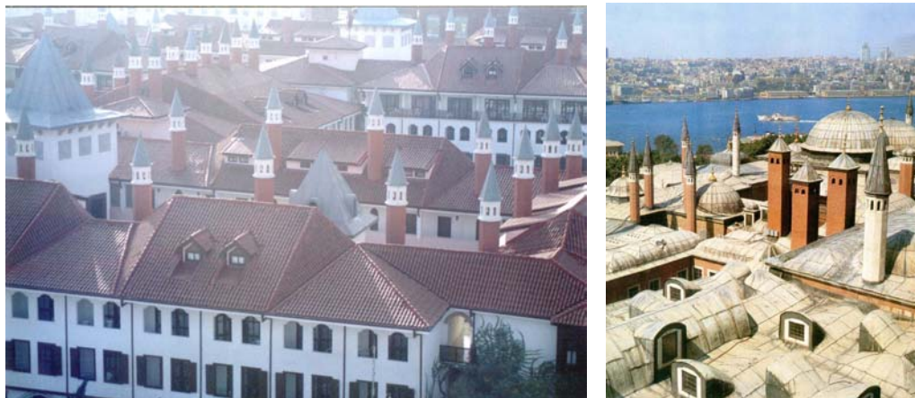
Figure 4.14 Guestroom blocks' roof on the left and Harem roof on the right (Akşit, 1993, p. 41).
