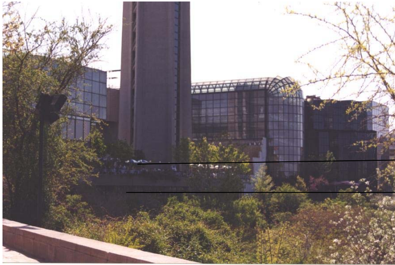
Figure 17 A photo taken (2003) from Çankaya caddesi showing the terraces with view to the park- upper open (featured by the author)
