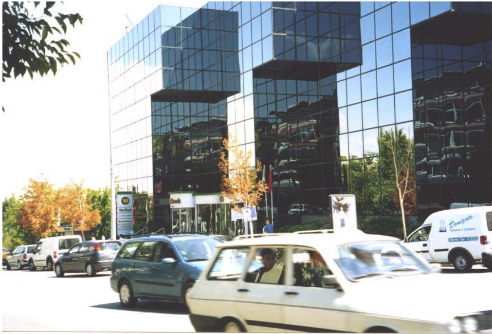
APPENDIX A. 7 taken from Cinnah Street showing Vakıfbank entrance-west elevation (2003).
