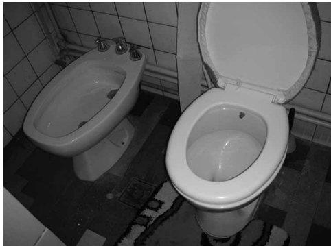
Figure 8. Bidet and alafranga lavatory in an un-renovated DHMİ Cooperative flat (photograph by the author, 2006).
