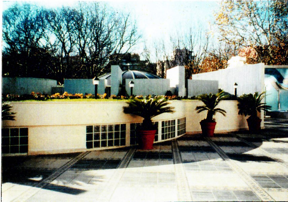
Figure 20. Roof of the gymnasium at Ceylan Intercontinental Hotel (November, 1996).
