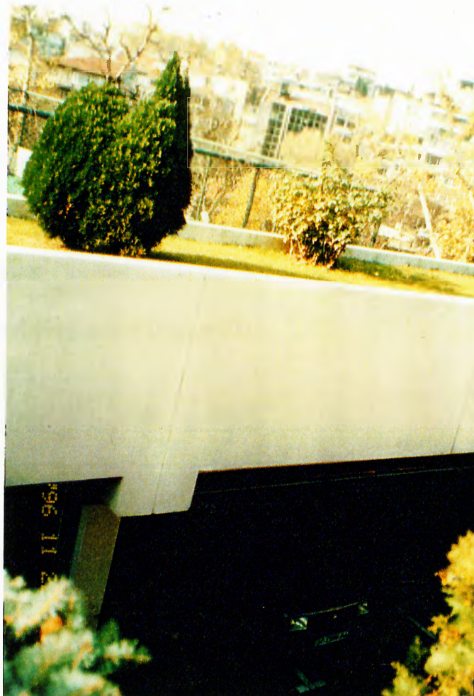
Figure 18. Roof of the underground garage at the Conrad Hotel (November, 1996).
