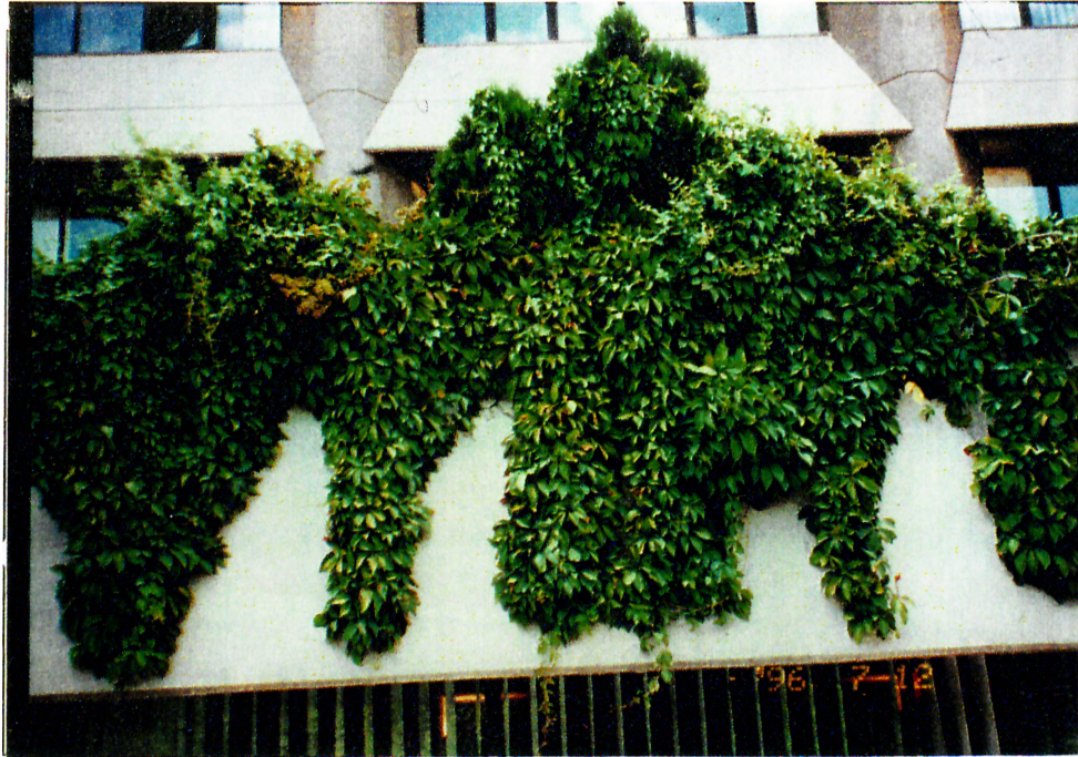
Figure 40. Plants, softening the contours of the Interbank Building (July, 1996).
