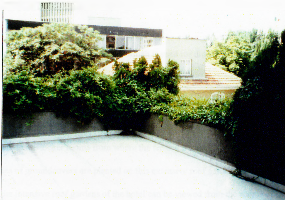
Figure 39. Roof garden on the second floor of the Interbank building (July, 1996).
