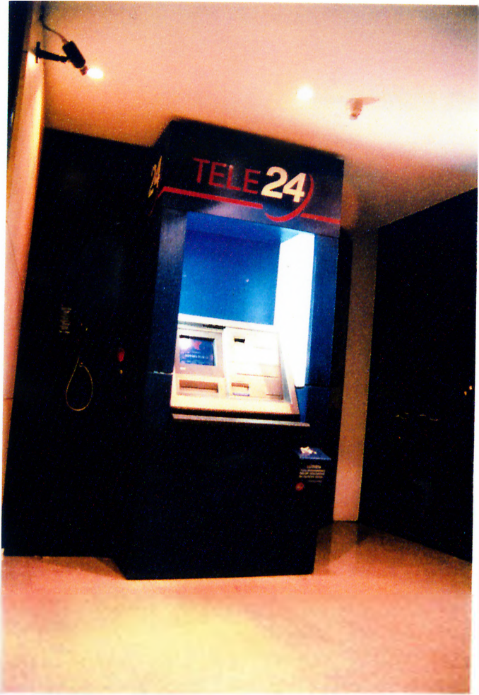
Figure A.3. View of the ATM Hall from Inside.
