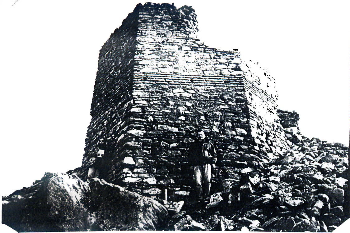
9 - T2 2nd phase (shell), from west.
