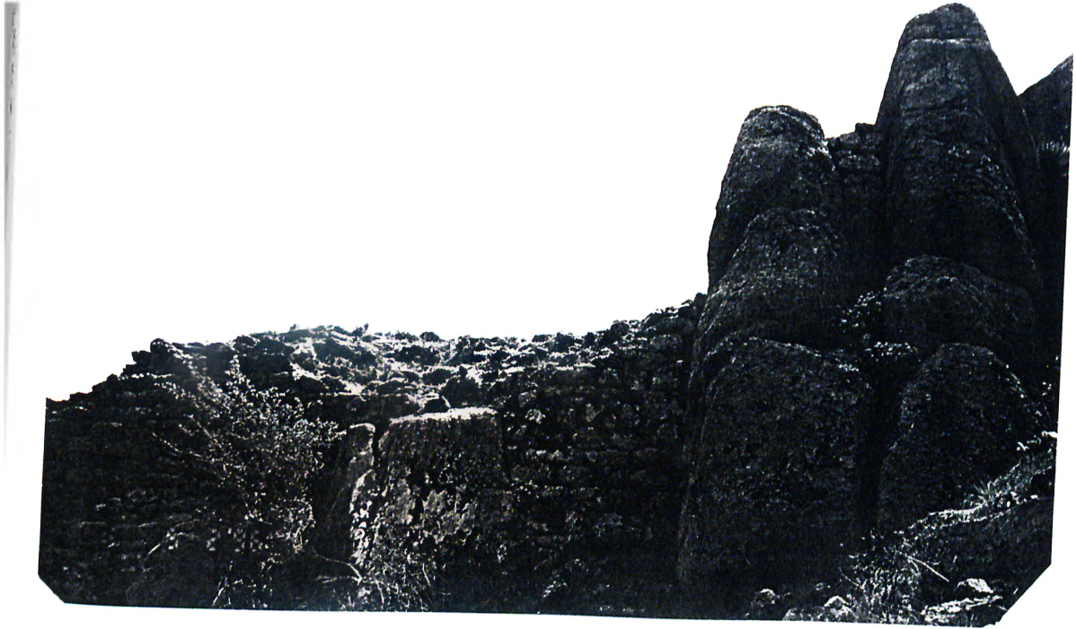
45 - Western end of the North Wall from north.
