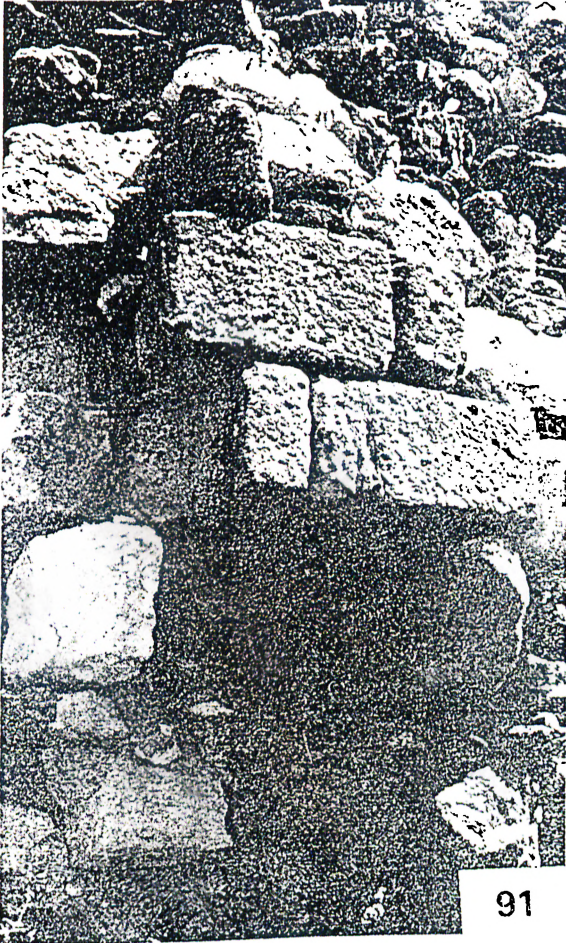
61 - Kayserkale, W1/2, detail of face, showing the carefully cut stonework of headers and stretchers (Foss 1985 fig. 91).
