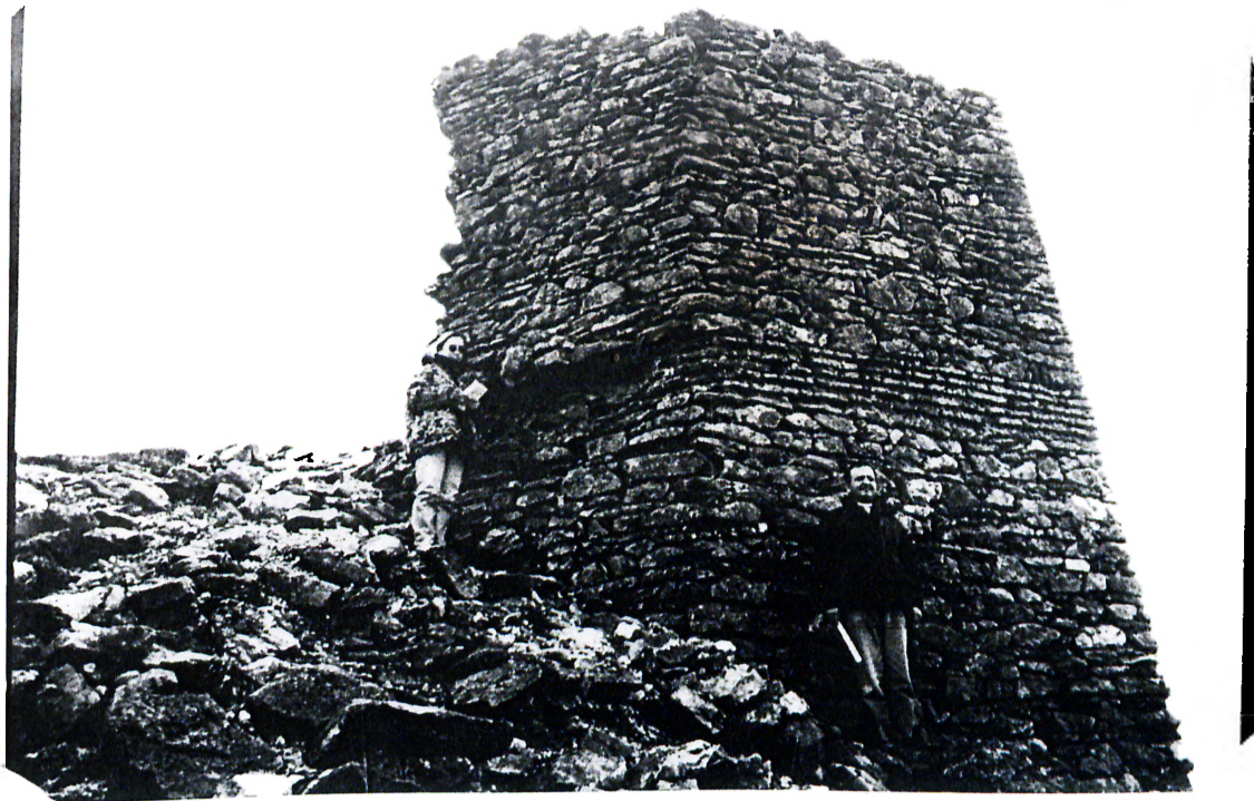
10 - T2 2nd phase (shell), from north.
