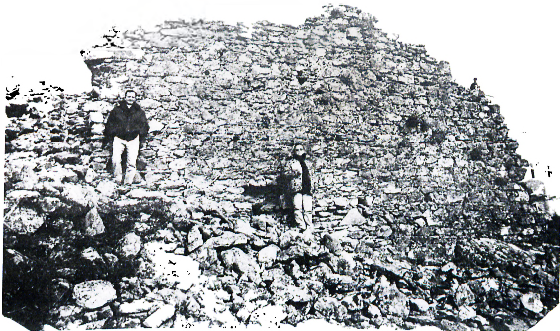
8 - T2 south wall.
