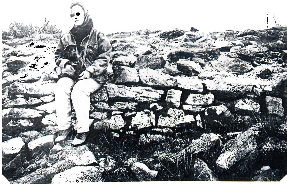
18 - T11 / T12 curtain outer facing.
