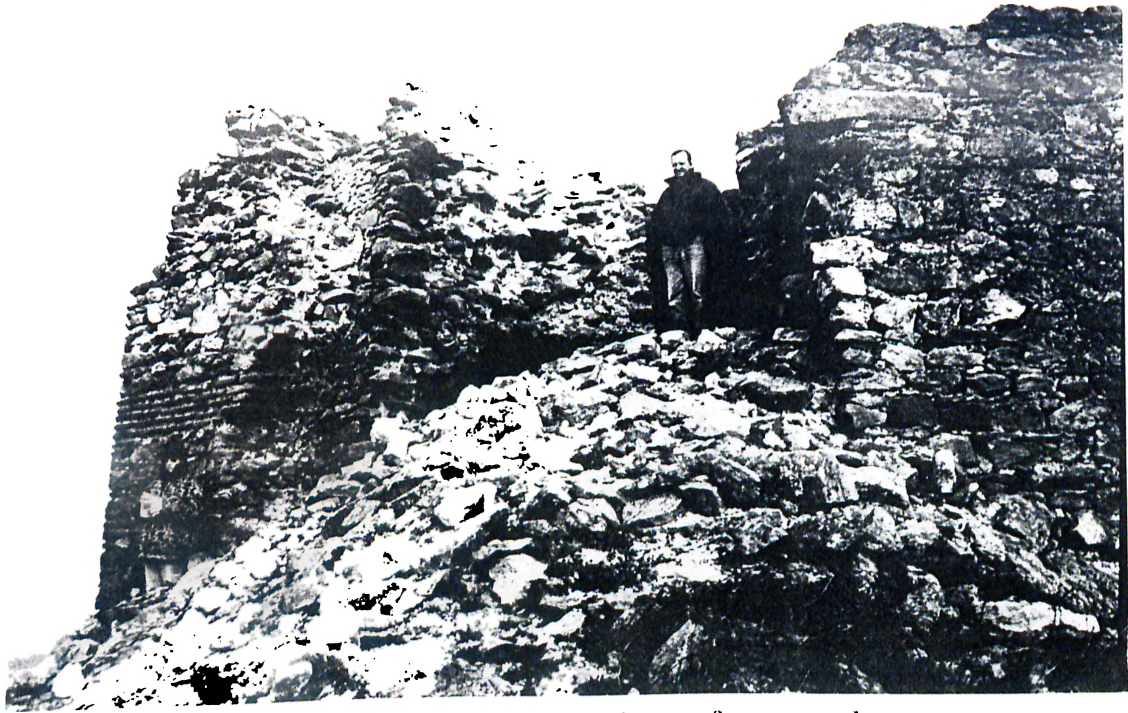
7 - T2 1st and 2nd phases from south west.
