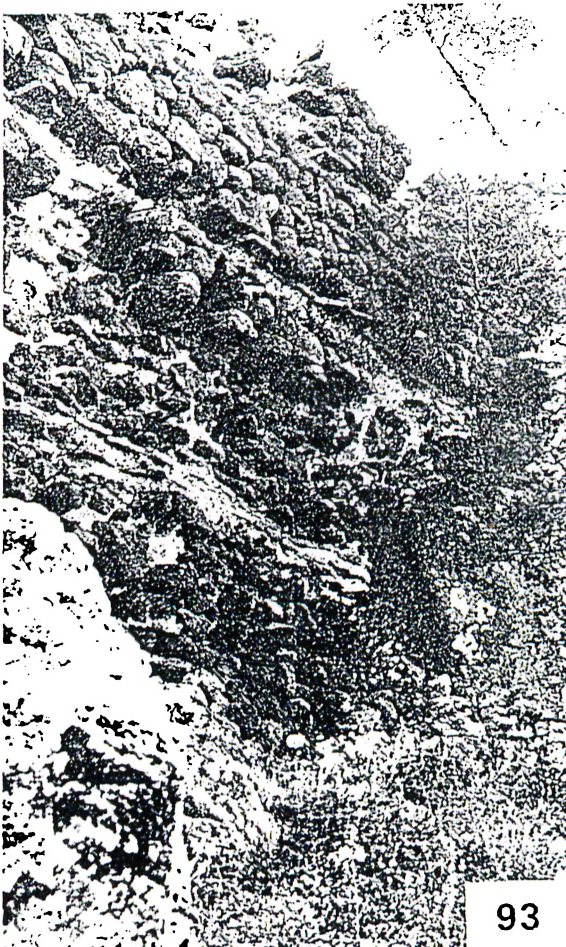
55 - Kayserkale, W2/3: masonry of coursed rubble with brick bands (Foss 1985 fig. 93).
