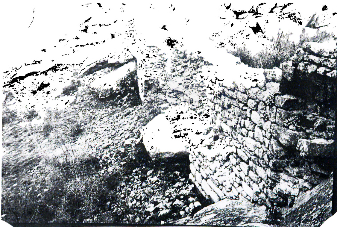
38 - T1, SW2 from south east.
