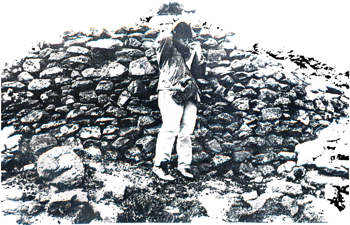
23 - T21 from south east.
