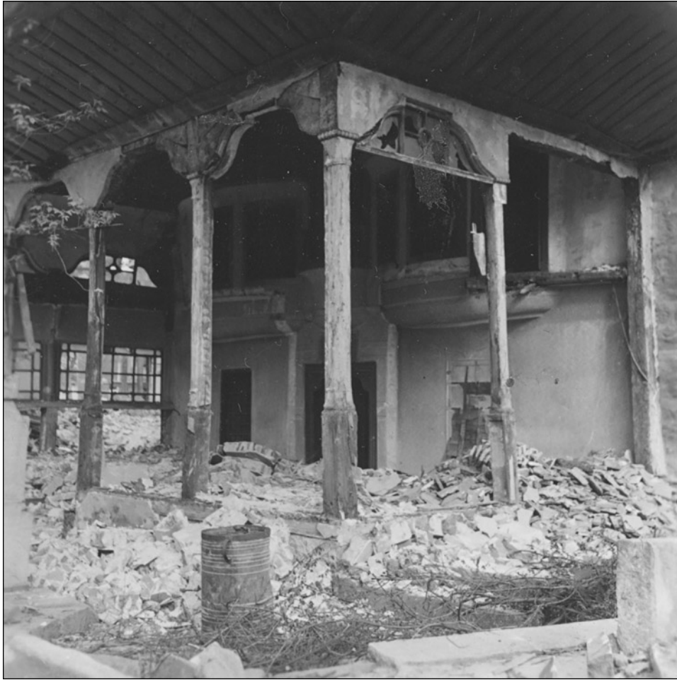
Fig. 63 Orta Mezar (Taşköprü) mosque, main entrance of the nineteenth century addition, view from NE (unknown photographer, 1968) State Archive Plovdiv
