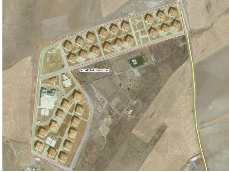
Figure 13: The aerial view of the blocks (www.googlemaps.com)
