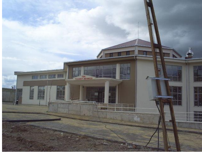
Figure 30: The vacant shopping center (Photograph by the author, 2012)
