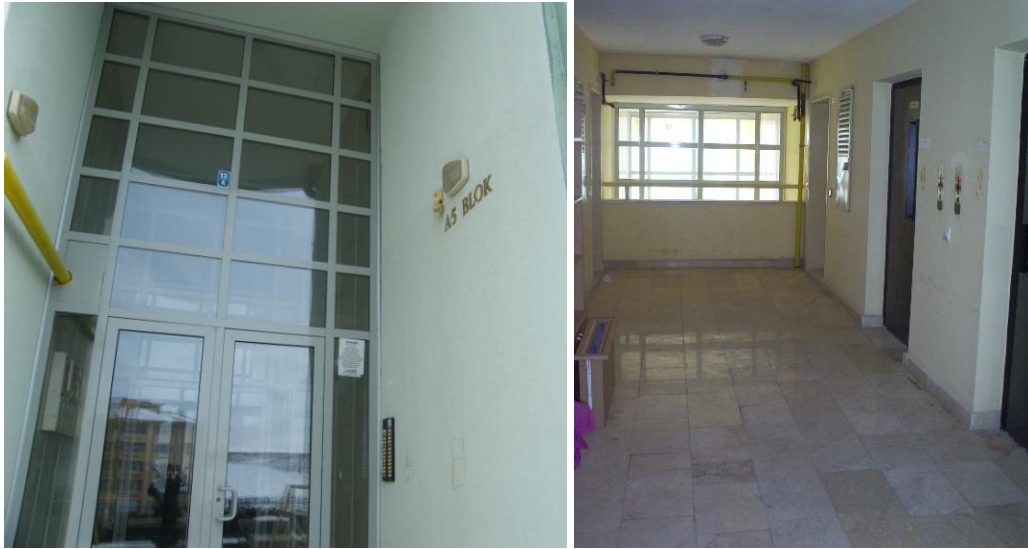
Figure 18 and 19: Entrance of a block and a view from the corridor of a block (Photograph by the author, 2012)
