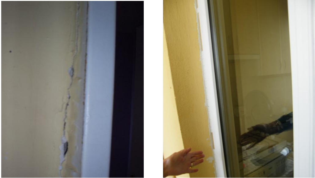
Figure 26 and 27: The cracks in the windows and doors (Photograph by the author, 2012)
