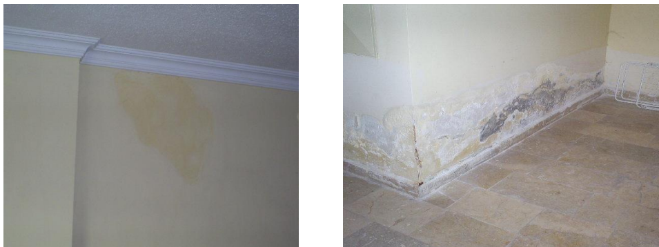
Figure 25: The damages in the finishing (Photograph by the author, 2012)
