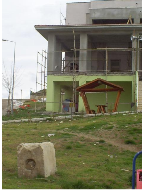
Figure 32: The unfinished construction work (Photograph by the author, 2012)
