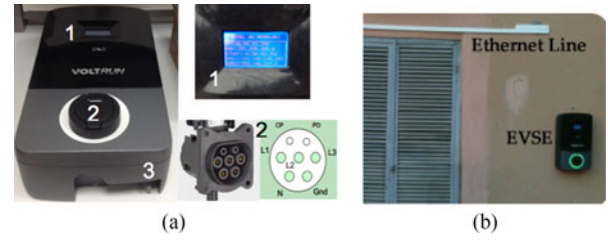
Fig. 11. Voltrun Mode 2 EVSE. (a) 1: IP settings for network connection, 2: IEC 61851 compatible charging socket, 3: ethernet connection port, (b) EVSE installation with Ethernet Line.
